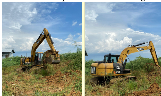
Gambar 5. Praktek pengoprasian Excavator
