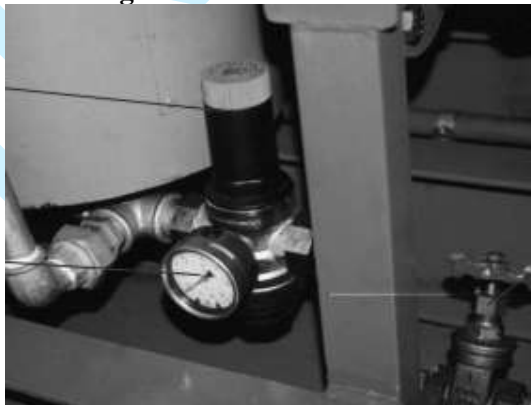
Gambar 3. Reducing Valve (sumber MT. Tirtasari)
