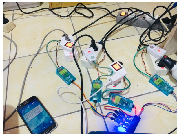
Figure 4 Electrical Load Measuring Device
