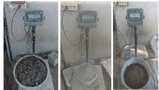
Gambar 7. Penimbangan Material Beton
