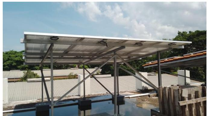
Figure 5. 3 kWp Solar Panel-1
