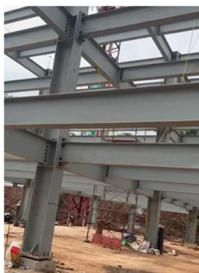
Figure 3. Connection with an additional horizontal plate to the weak axis of the column Source: Adapted from [4]
